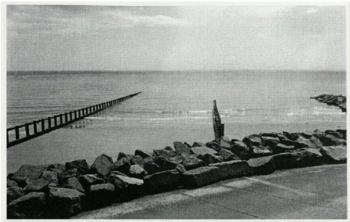
(Figure 7.7) Felpham foreshore looking almost north across the near-shore part of the area of Bed 3, including the lignite bed and the channel infill, and showing new sea defences in foreground and at right. In this photograph most of the strata are underwater or are covered by modern beach deposits. Taken in 1999. (Photo: M.E. Collinson.)
