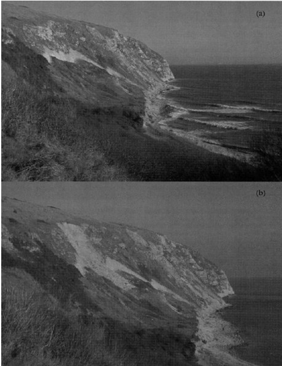
(Figure 4.30) Ballard Down. Views looking east from [SZ 038 810] (a) taken on 12 January 2001 and (b) on 16 January 2001, showing the development of the landslide over four days. In (a) note the chalk scar formed by the failure of the slope. In (b), note the rectangular scar of the shallow rockslide that followed removal of bedrock and weathered slope materials at the back of the earlier failure. (Photo: V.J. May.)
