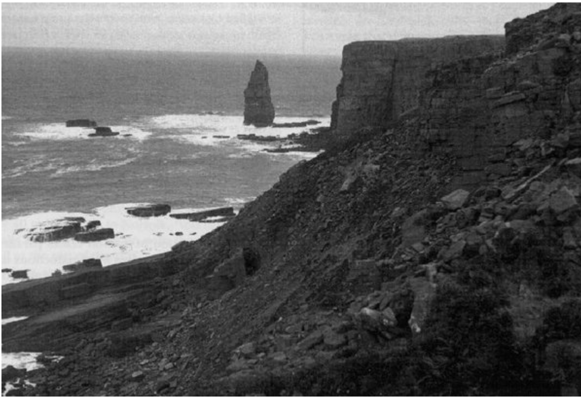
(Figure 2.4) Toppling in the Torridonian sandstone cliffs south of Sandwood Bay, Sutherland. Dipping beds of well-jointed sandstones are subject to subaerial weathering and failure. Strong surf prohibits the debris from accumulating at the cliff foot. The stack in the distance is Am Buachaille (Gaelic for 'herdsman'). (Photo: J.D. Hansom.)
