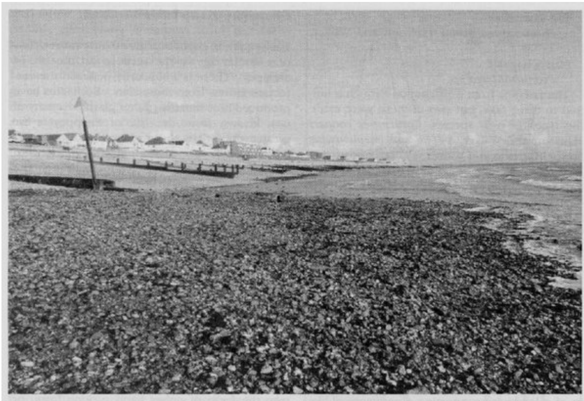
(Figure 4.12) General view of the Lee-on-the-Solent GCR site, which provides foreshore exposures of Middle Eocene sediments, one of the very few Middle Eocene fossil bird localities. (Photo: Dave Evans.)
