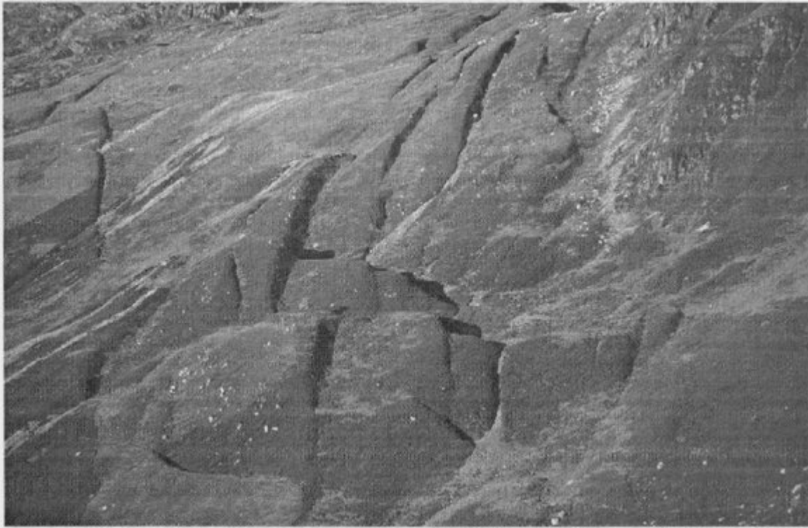
(Figure 2.45) Close-up of the Beinn Each rock slope failure nexus, suggesting extrusion of a component of the failed mass with fracturing along two joint-sets. (Photo: D. Jarman.)
