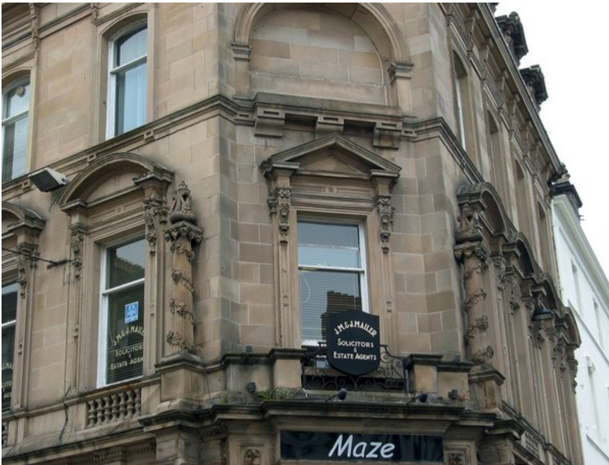
(Plate 1.1) Locality 1.8. Corner of Murray Place and King Street, former Bank of Scotland; Upper Limestone Formation sandstone from Polmaise Quarry.
