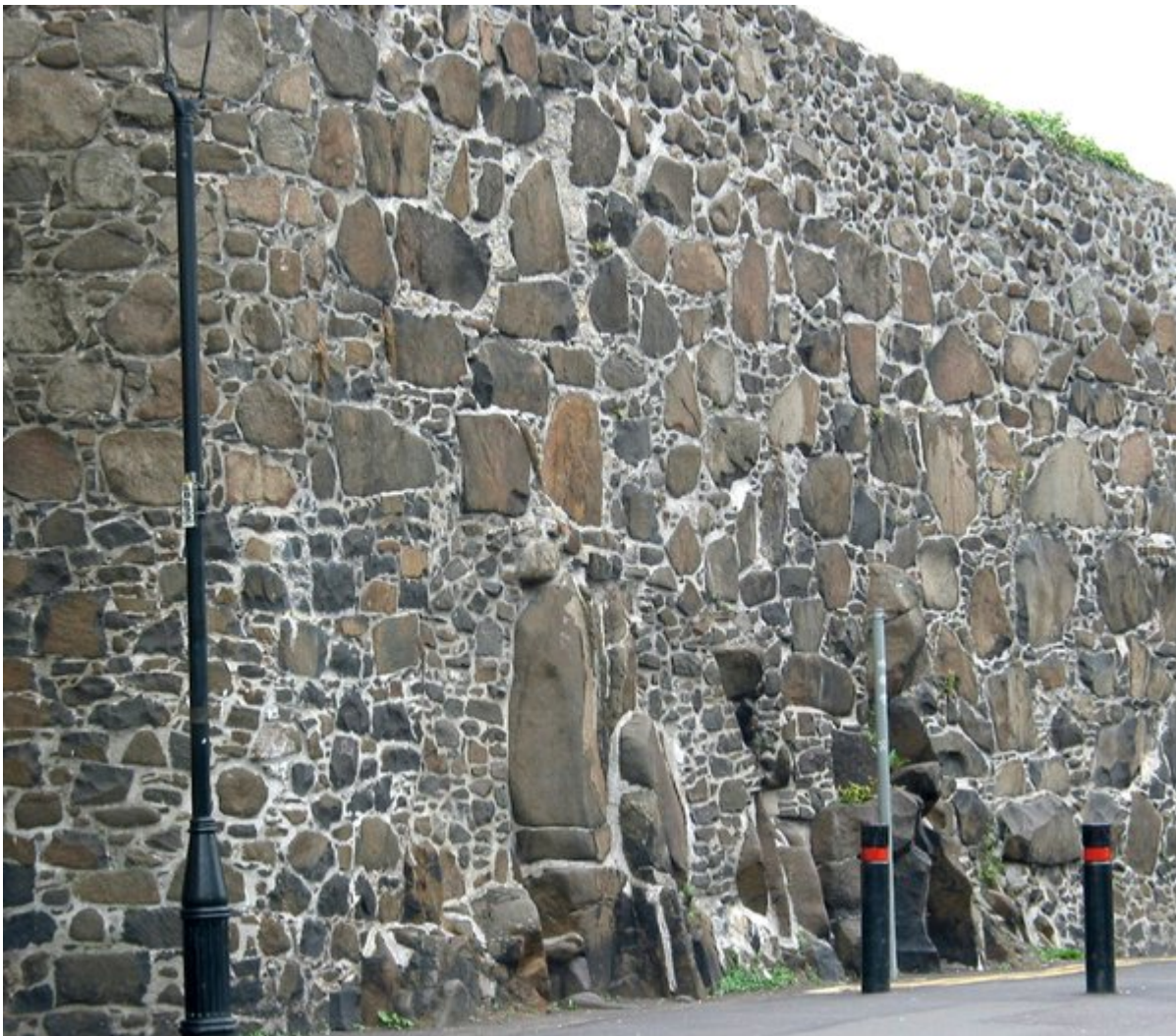
(Plate 1.3) Locality 1.13. City wall at Back Walk in blocks of local quartz-dolerite. Bedrock of same quartz-dolerite seen at pavement level.
