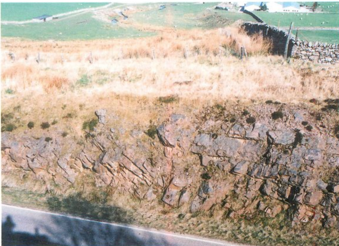
(Figure 4.3) Ousdale road cutting on the A9 (north end, southbound side) showing the junction between sheared granite and bedded arkose. (Locality now more overgrown with vegetation.)
