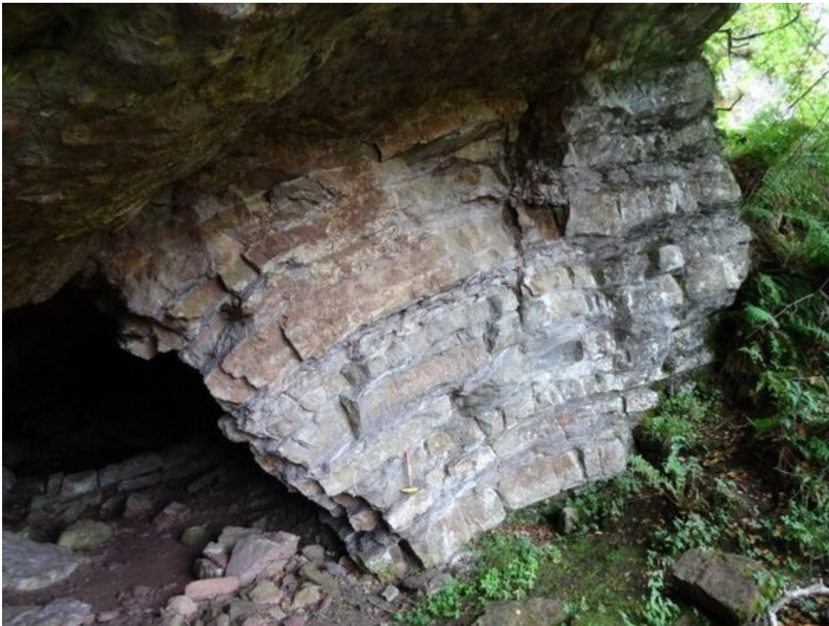
(Figure 6) Post of limestone supporting the roof of the limestone mine at Locality 8. The roof of the mine is studded with Gigantoproductus shells.
