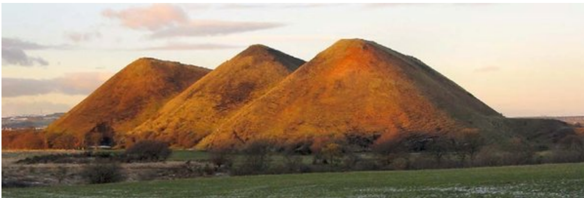
(Figure 27) Five Sisters oil-shale bings [NT 009 641] (WLGS 5) from the south. Burnt oil-shale is initially dark blue-grey ("blaes"), but rapidly oxidises to a characteristic red colour in contact with the elements.
