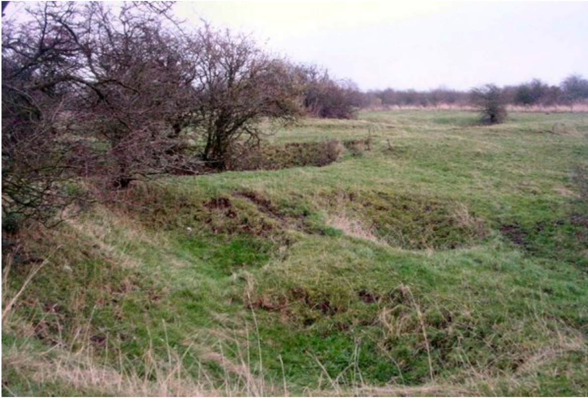
(Figure 37) Sitts resulting from the collapse of underground stope and room working. Upper Uphall [NT 0550 7225] (WLGS 11). Hopetoun Member, West Lothian Oil Shale formation.
