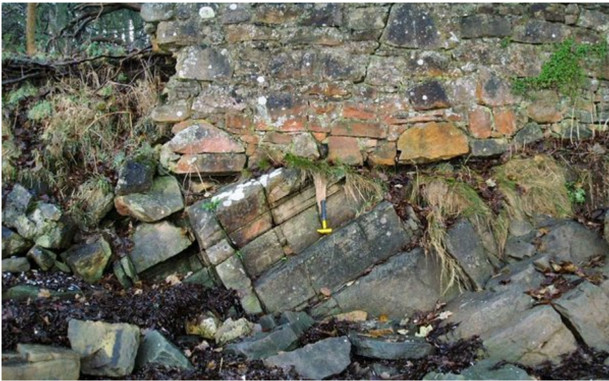
(Figure 52) Blending in — wall of local sandstone built on eastward-dipping Dunnet Sandstone at Society Shore 2 [NT 0954 7913] (WLGS 16). Hopetoun Member, West Lothian Oil Shale Formation.
