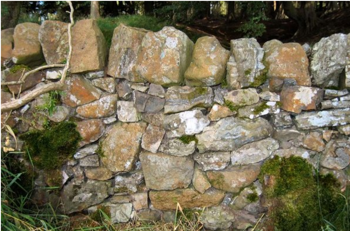
(Figure 73) Drystone dyke of Wairdlaw Limestone at Wairdlaw Quarry [NS 9952 7313] (WLGS 21).
