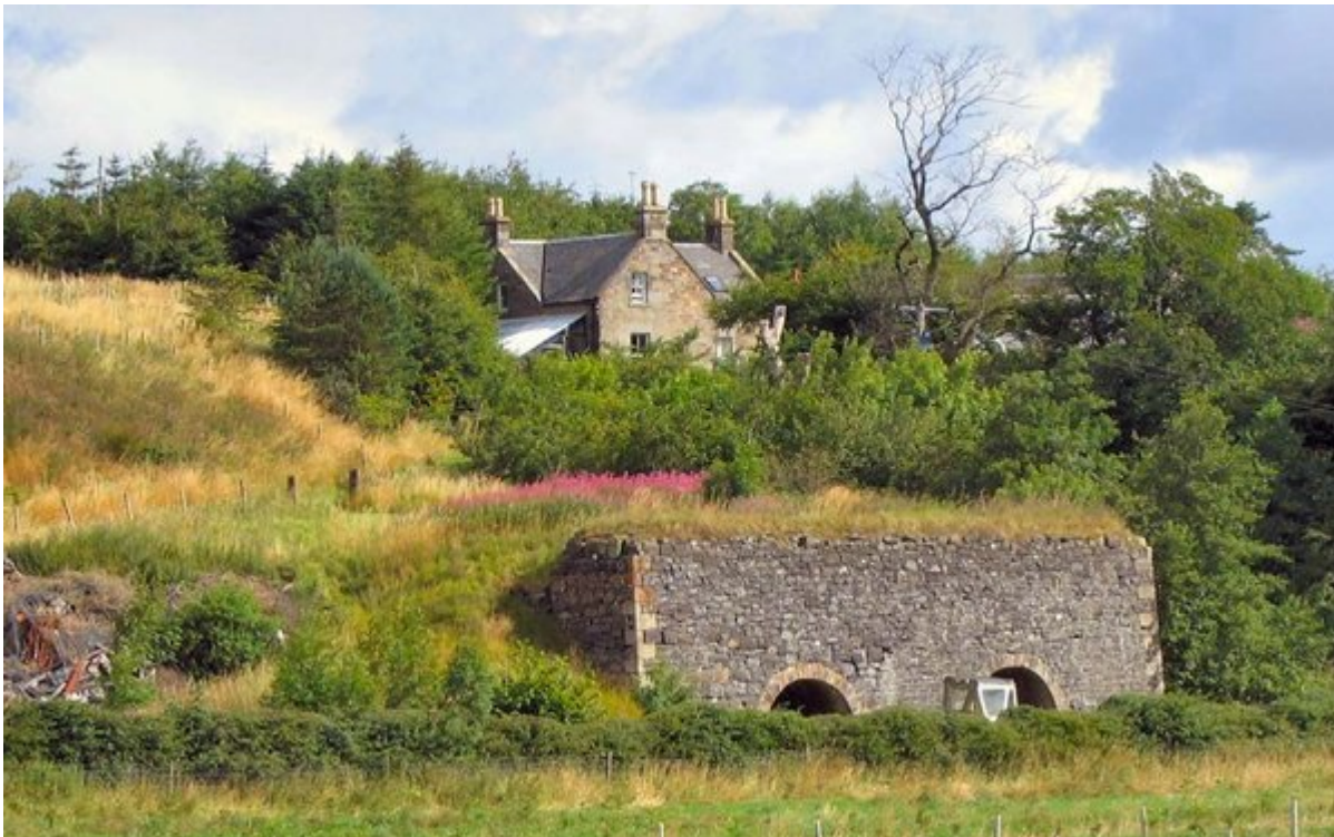
(Figure 69) Well-preserved lime kilns at Wairdlaw Quarry [NS 9955 7304] (WLGS 21).
