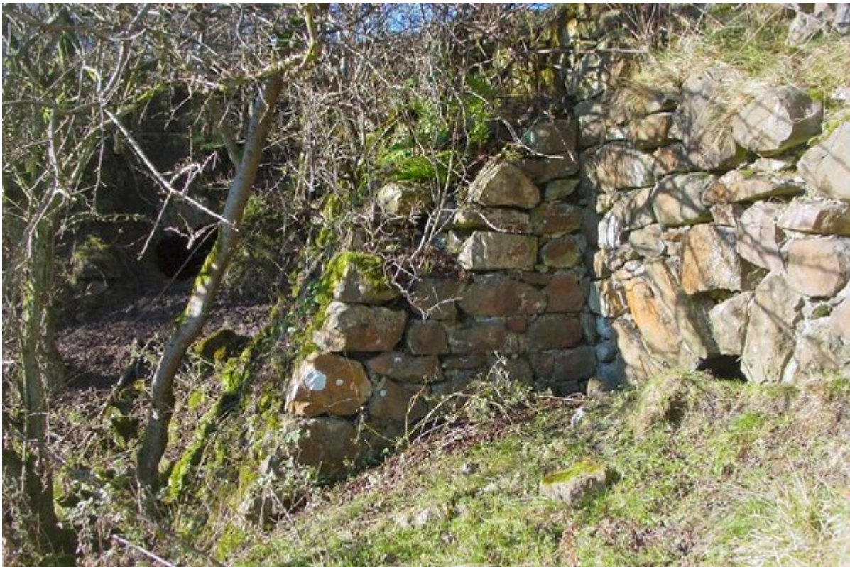
(Figure 100) Lead-Zinc mine adit at Hilderston Silver Mine [NS 9917 7158] (WLGS 29).
