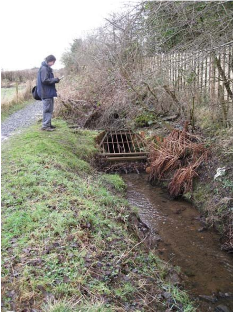
(Photo 37) Craigdhu Burn channelled underground. Looking SE.
