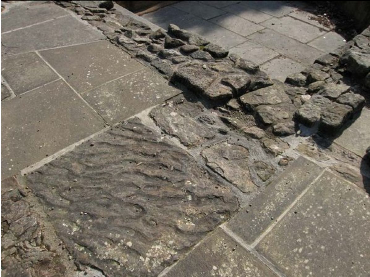
(Photo 144) Close-up of the original flagstone paving at the Roman bath-house, which displays fossilised ripples.
