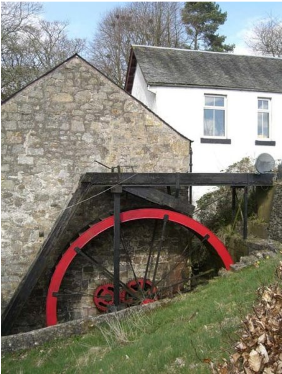
(Photo 177) Baldernock Mill, built from local sandstone during the 16th century, included a brick kiln in the basement for drying the grain before milling. The present wheel, seen above, is 18ft in diameter with 48 steel buckets.
