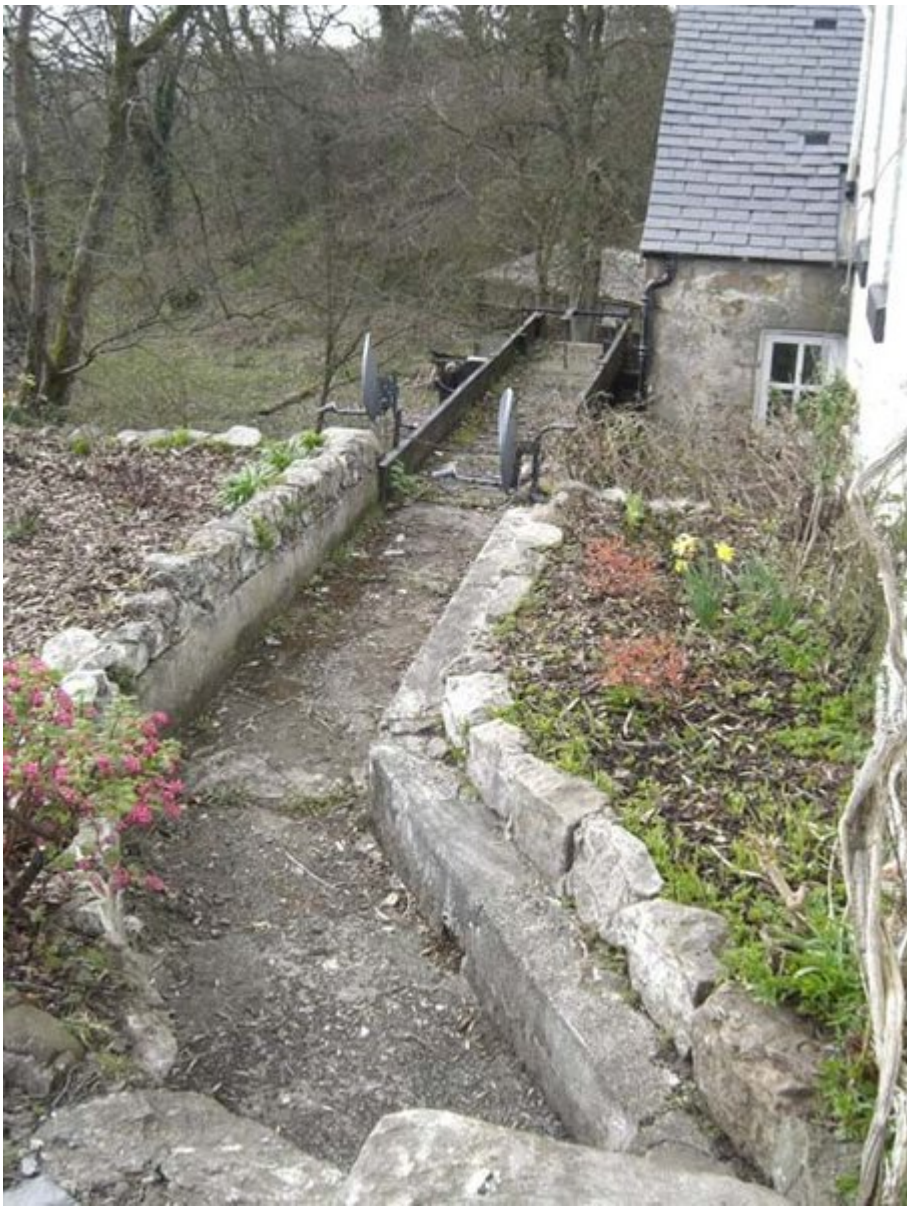
(Photo 178) The water supply for Baldernock Mill came from a dam 250yds upstream; running through a tunnel beneath the road to reach the mill, seen above. The mill was largely restored in the 1970's after falling into disrepair.
