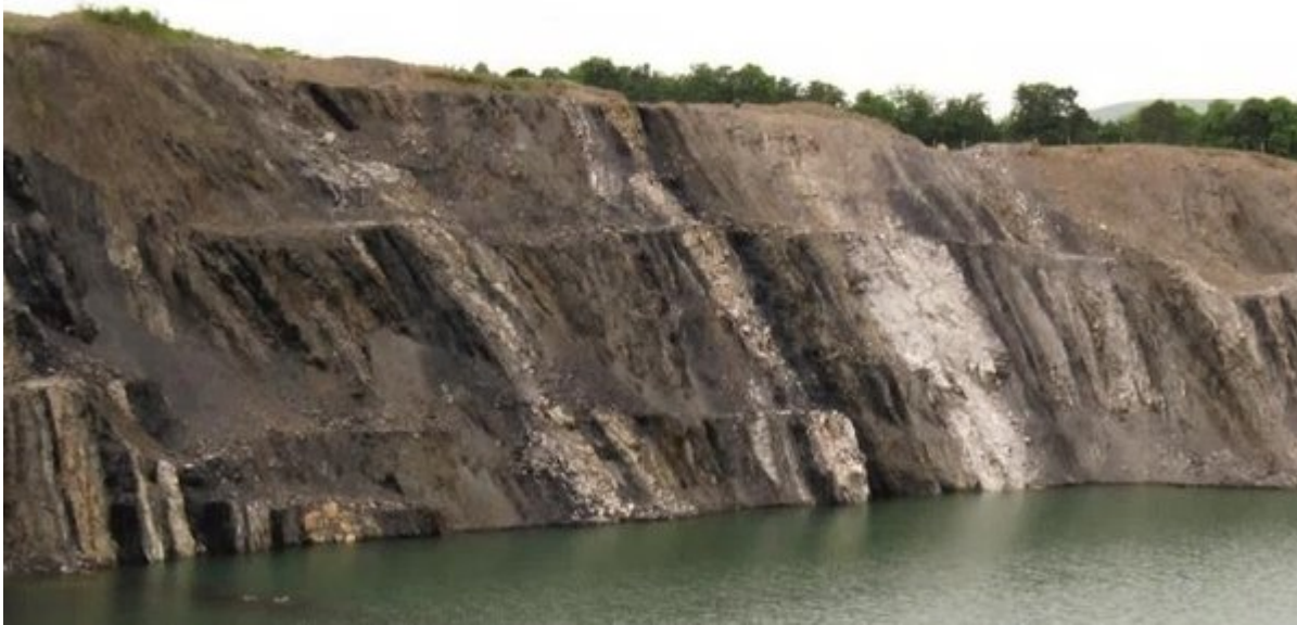
(Figure 12) Main face of Mainshill Wood SCM showing the sub-vertical strata. The darker layers visible in the mined face are coal seams (the Manson Coals in the centre of the image), whilst the lighter layers are sandstones and limestones. Note high water level restricting access to base of exposures. Photo taken June 2014. © BGS, NERC
