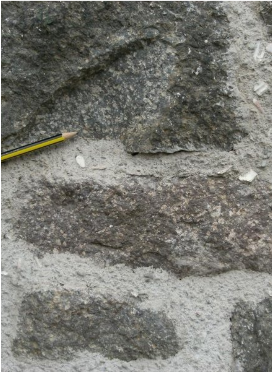
(ELC_12_P3) Close-up of porphyritic trachyte blocks used in the John Gray Centre. Note the large pale-coloured crystals (phenocrysts) scattered within a fine-grained dark green/purple groundmass. Typical of the material seen in Peppercraigs Quarry. © BGS, NERC.
