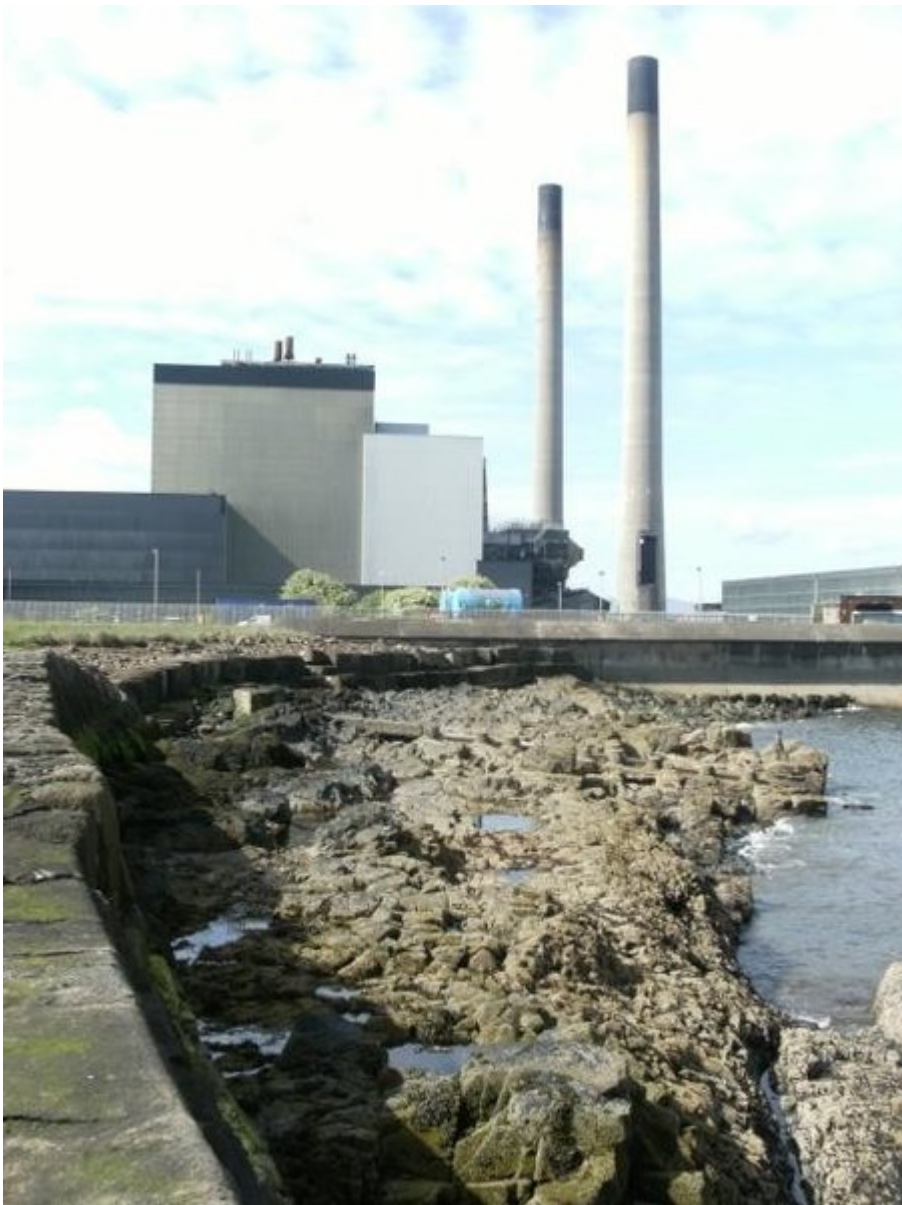
(ELC_16_P1) Cockenzie Power Station, looking west. The rocks in the foreground are the igneous rocks of the Port Seton-Spittal Dyke. © BGS, NERC.
