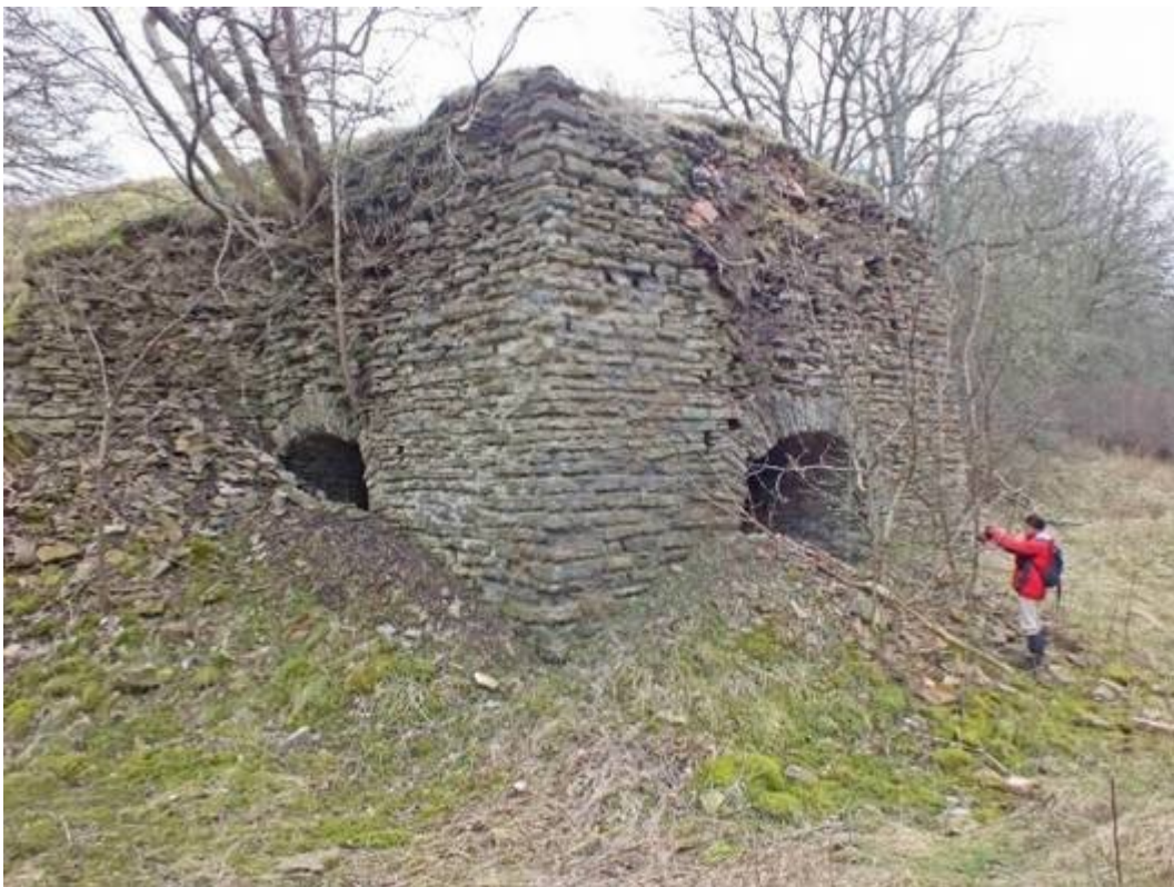
(Figure 5) SP 2. Currie Lee Limestone Quarries. SP 3. Lime Kiln at [NT 3795 6205].
