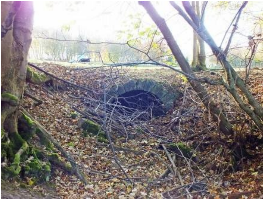
(Figure 34) SP 30. Arch over a shallow trench. A former waggonway for hauling lime down to Mayfield and beyond. [NT 3519 6335].
