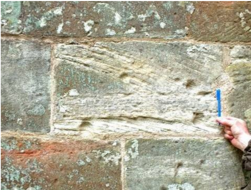
(Figure 6) SP 4. Crichton Kirk. [NT 3811 6161]. Geologically, this block is laid upside-down: the first layers deposited are at the top of the block, and were laid down at an angle. Then the tops of these layers were eroded before the second set of layers were laid down horizontally
