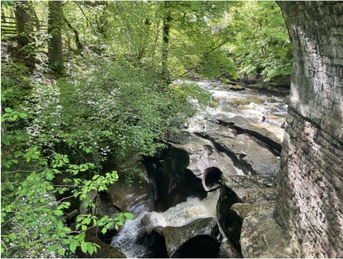
(Photo 09-1) The "Span of Eden" eroded in the Brockram beneath Stenkrith Bridge.
