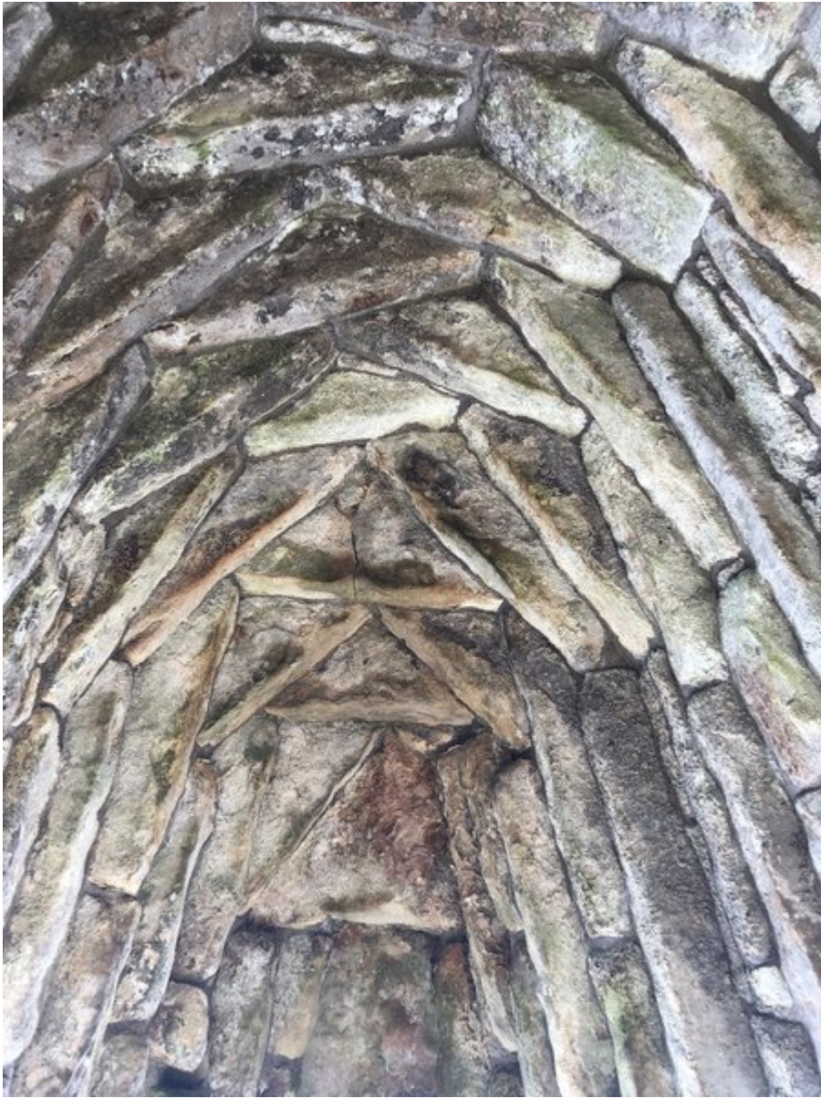
(Photo 00-3) Ceiling at Crindledykes limekiln.
