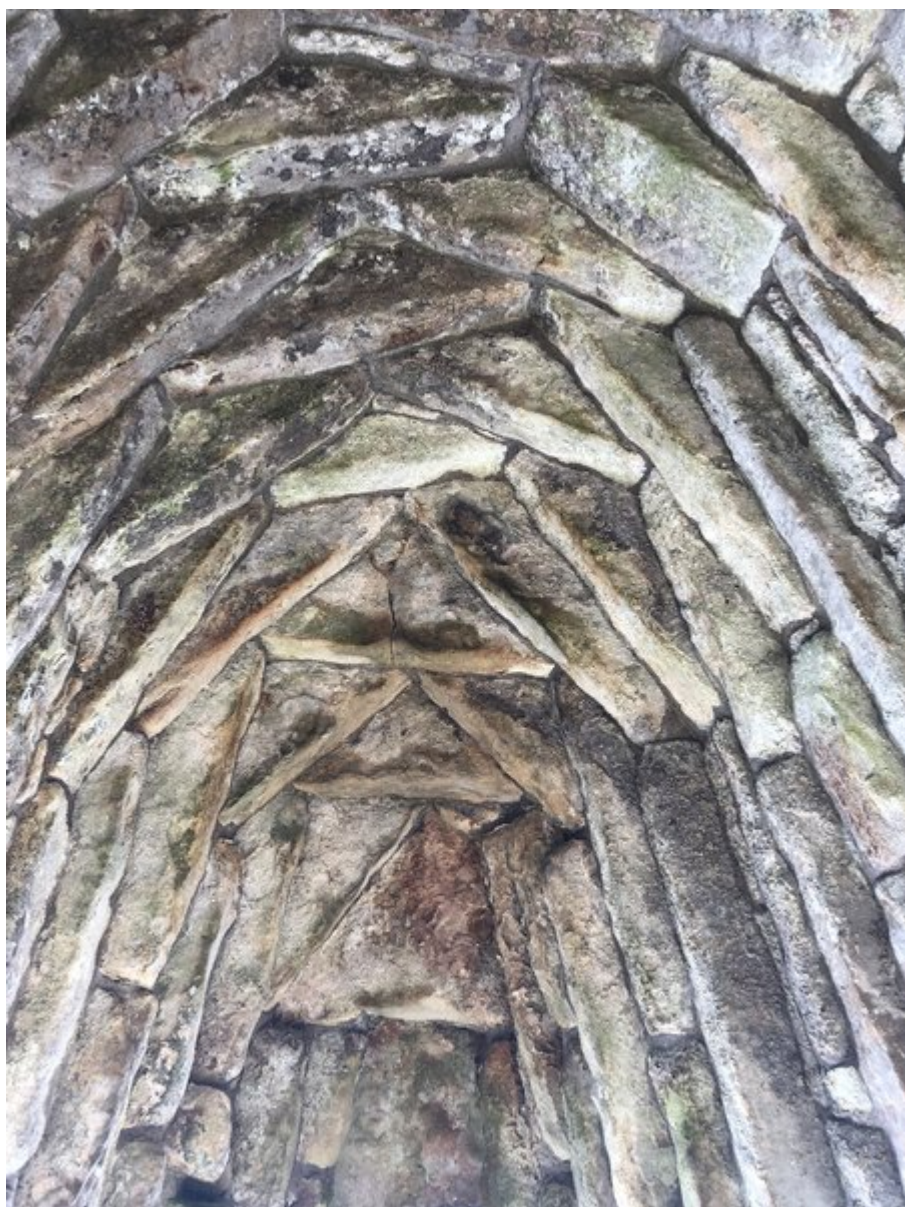
(Photo 00-3) Ceiling at Crindledykes limekiln.
