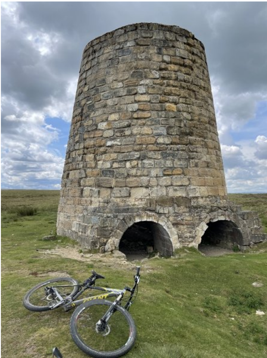
(Photo 38-1) Smelt mill chimney, Allenheads.
