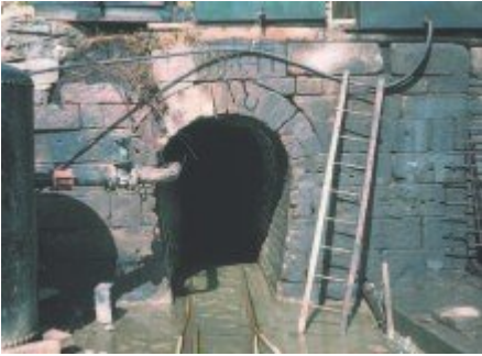
(Photo 78) Cambokeels Mine, Weardale. The original stone-arched horse level. B Young, BGS, ©NERC, 2004.
