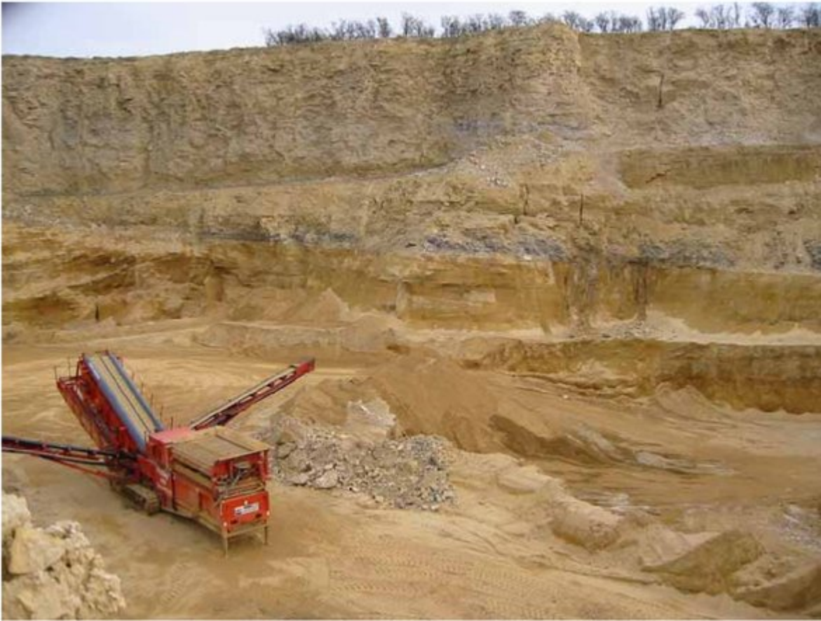
(Plate 21) Magnesian Limestone (Raisby Formation) overlying the Marl Slate Formation (the grey layer) above the Yellow Sands Formation in the working Hepplewhites Quarry.
