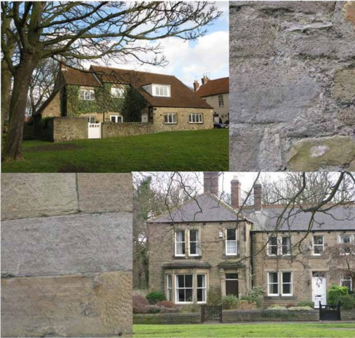
(Plate 18) Use of magnesian limestone as building stone in Whitburn.
