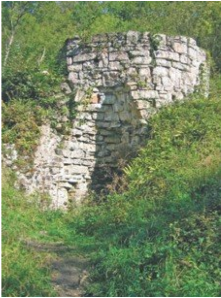
(Figure 16) Recently restored limekiln, Vallis Vale.
