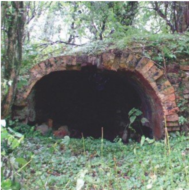
(Figure 39) The remains of a bank of coking ovens, Vobster Breach Colliery.
