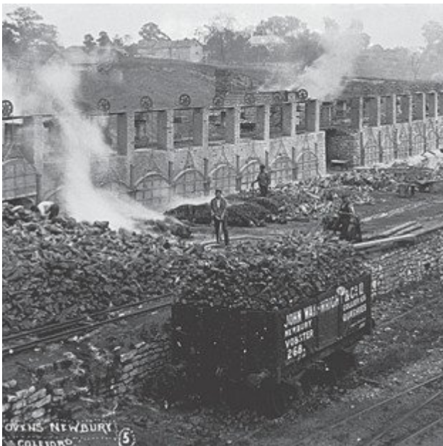
(Figure 36) Wainwright's Newbury Colliery showing the extensive coke ovens and some of Wainwright's privately owned rail wagons. Courtesy of the John Cornwell collection.
