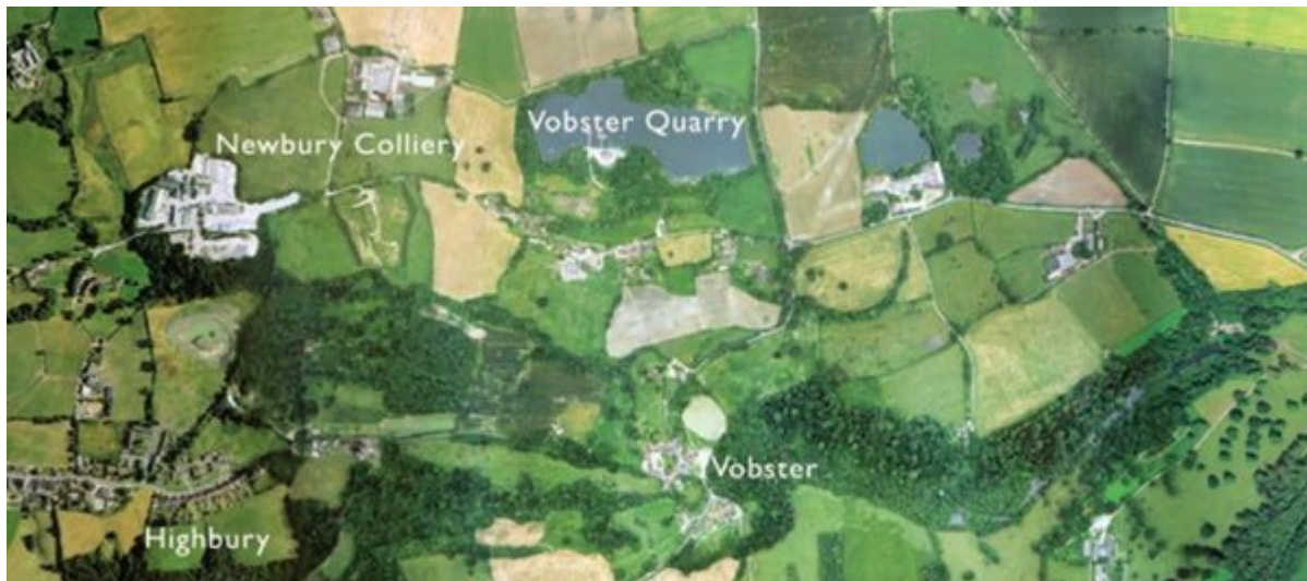
(Figure 34) Aerial photograph of the Vobster area.
