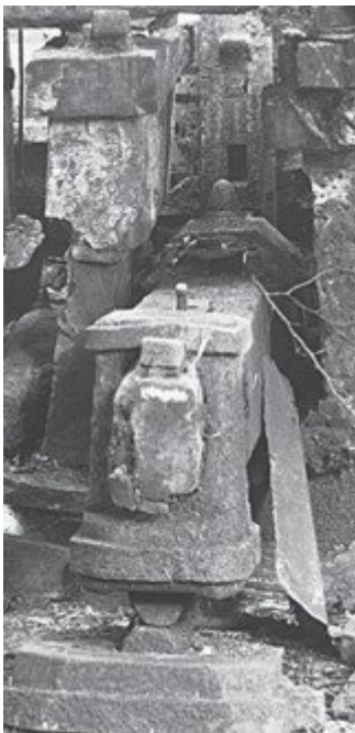
(Figure 63) Gurney Slade Forge, with tilt hammer. Dr P R Reid, 1933. Courtesy of the John Cornwell collection.
