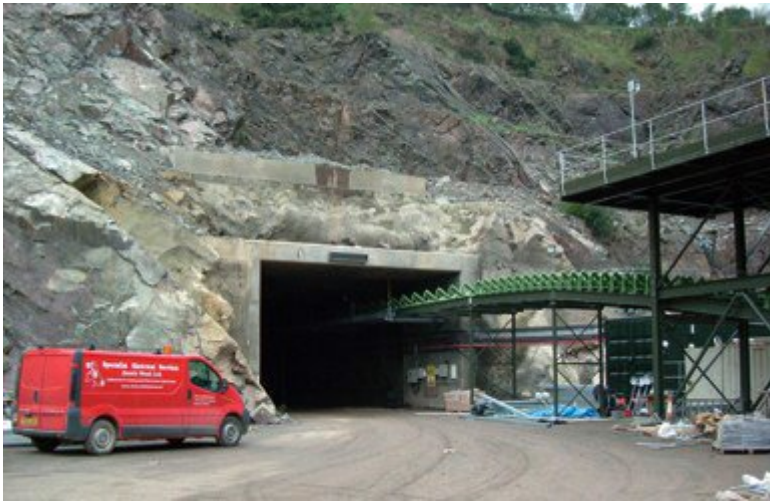
Tunnel linking the two Cliffe Hill quarries.
