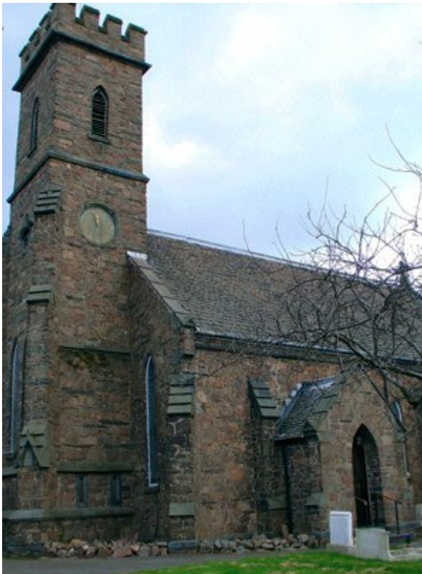
Groby Church with its Swithland Slate roof and local Charnian rocks in the walls.
