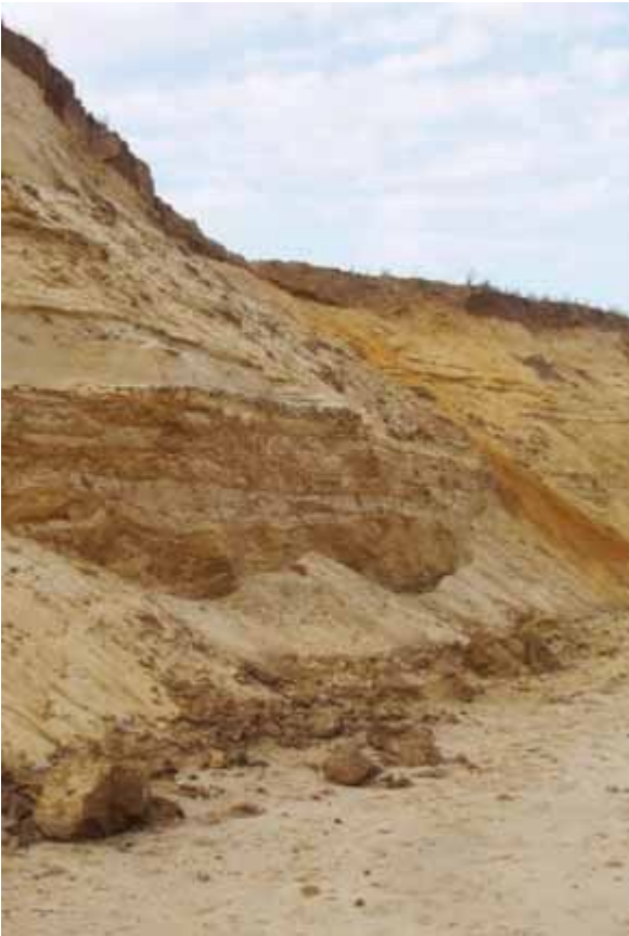
Sands, gravels and clays of the Norwich Crag formation exposed in Covehithe Cliffs. Similar deposits are forming offshore at the present day.
