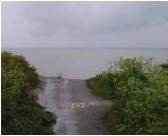
Road to nowhere. Visitors may see old wartime drain pipes, electricity cables and bundles of barbed wire eroding out of the cliffs. Recently a concrete pillbox was swallowed by the sea.
