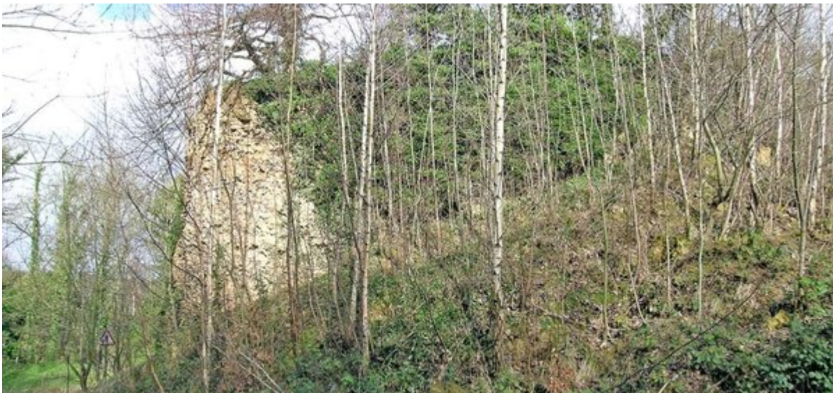
(Figure 92) General view of south face of breccia stump. [SE 53457 00488].
