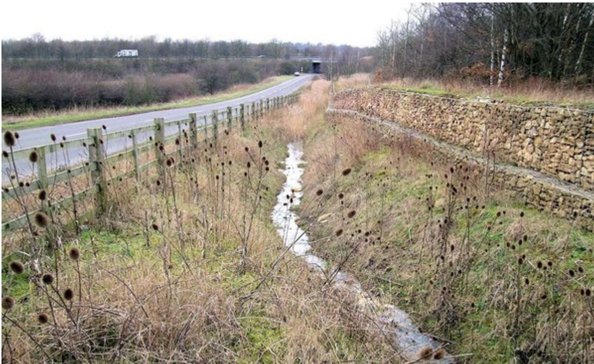
(Figure 124) General view along drainage ditch to the west. [SE 52340 06650].
