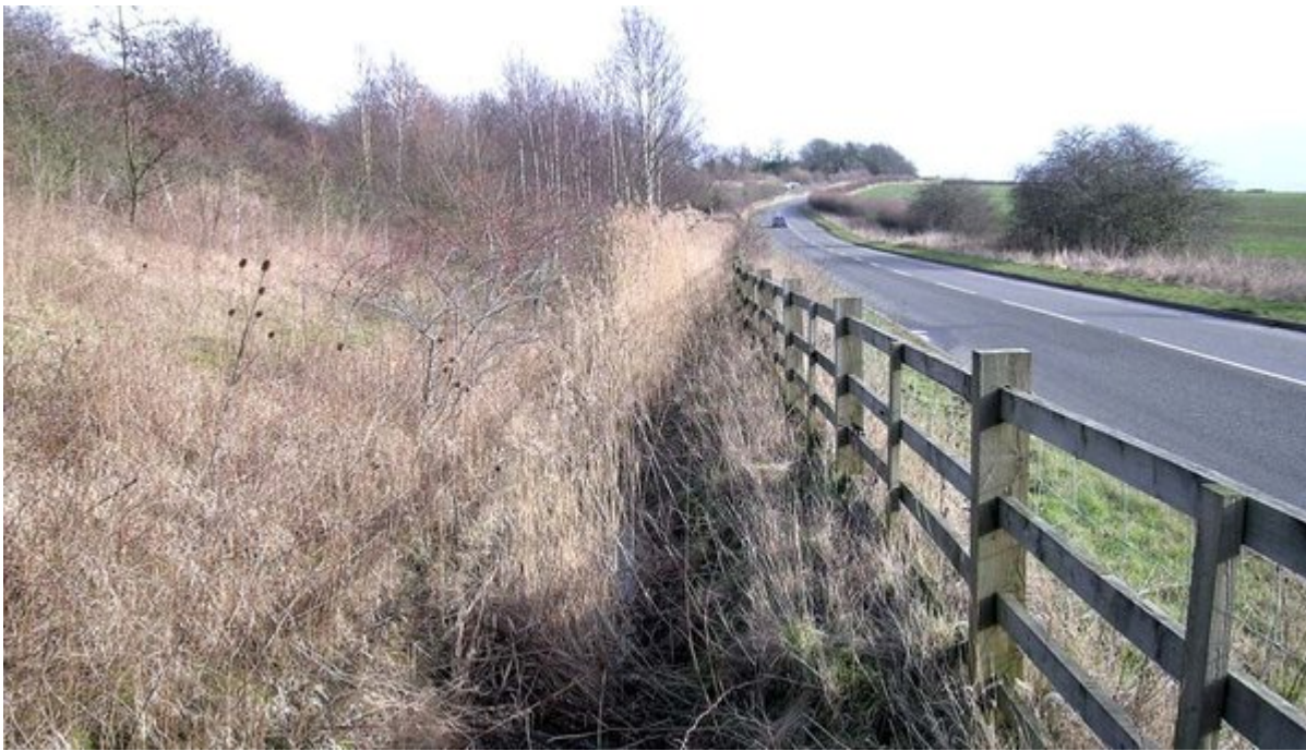
(Figure 123) General view along drainage ditch to the east. [SE 52150 06720].
