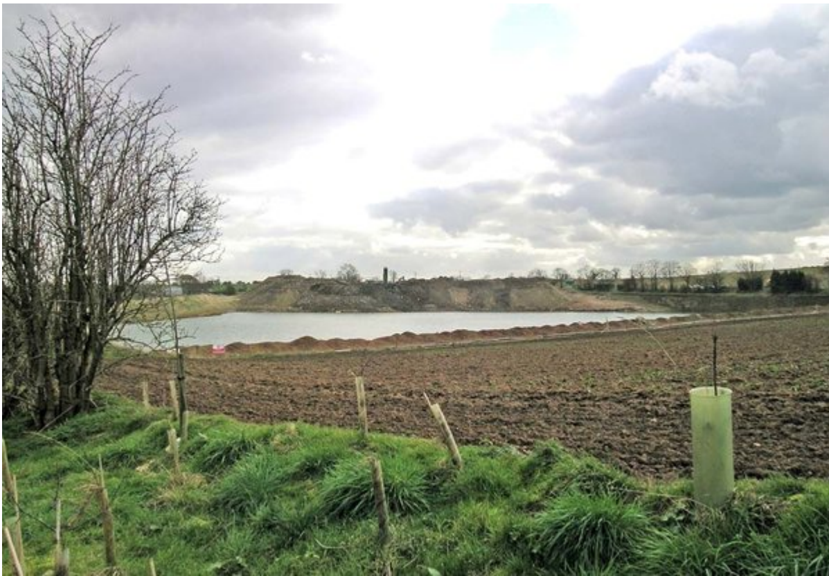
(Figure 134) General view of restoration and tree planting works. [SE 51116 11573].
