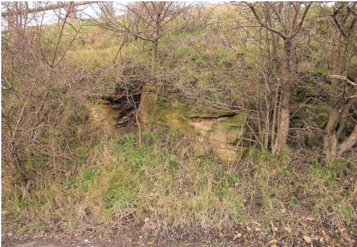
(Figure 15) Road cutting exposure of Mexborough Rock with vegetation overgrowth.[SK 48974 99510].
