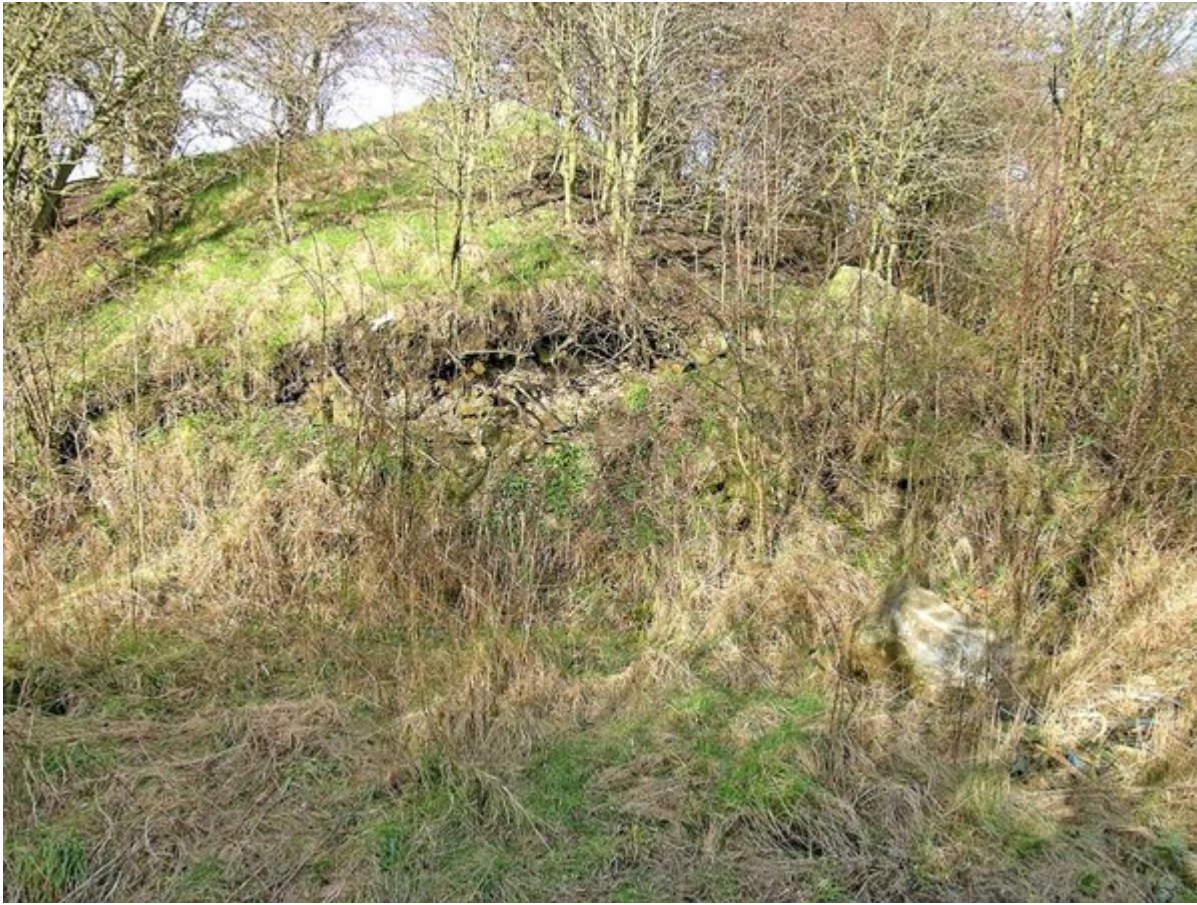
(Figure 24) Exposure A. Massive Ackworth Rock overlain by flaggy rock and soil in embankment. [SE 47721 03309].
