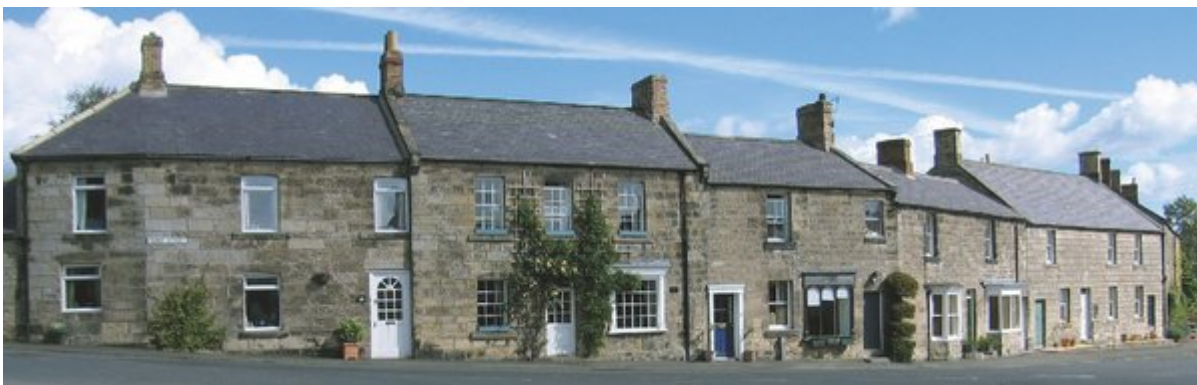
(Figure 72) Houses built from local sandstone in Front Street, Glanton.
