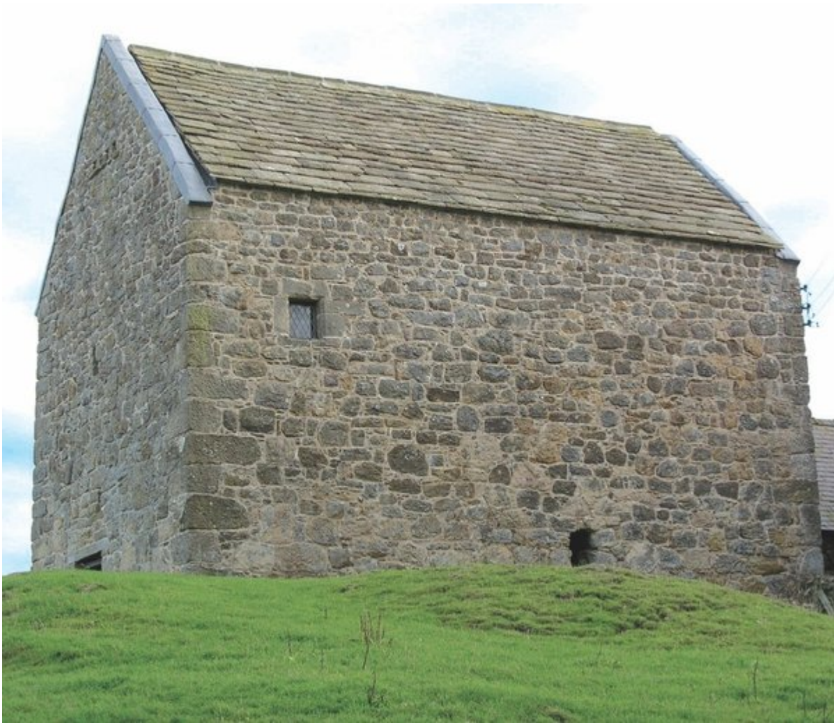
(Figure 74) Hole Bastle, near Bellingham, constructed from random rubble sandstone with roughly dressed larger blocks used for corner stones and surrounds to openings. The flagstone roof is typical of those once common in southern parts of the district.
