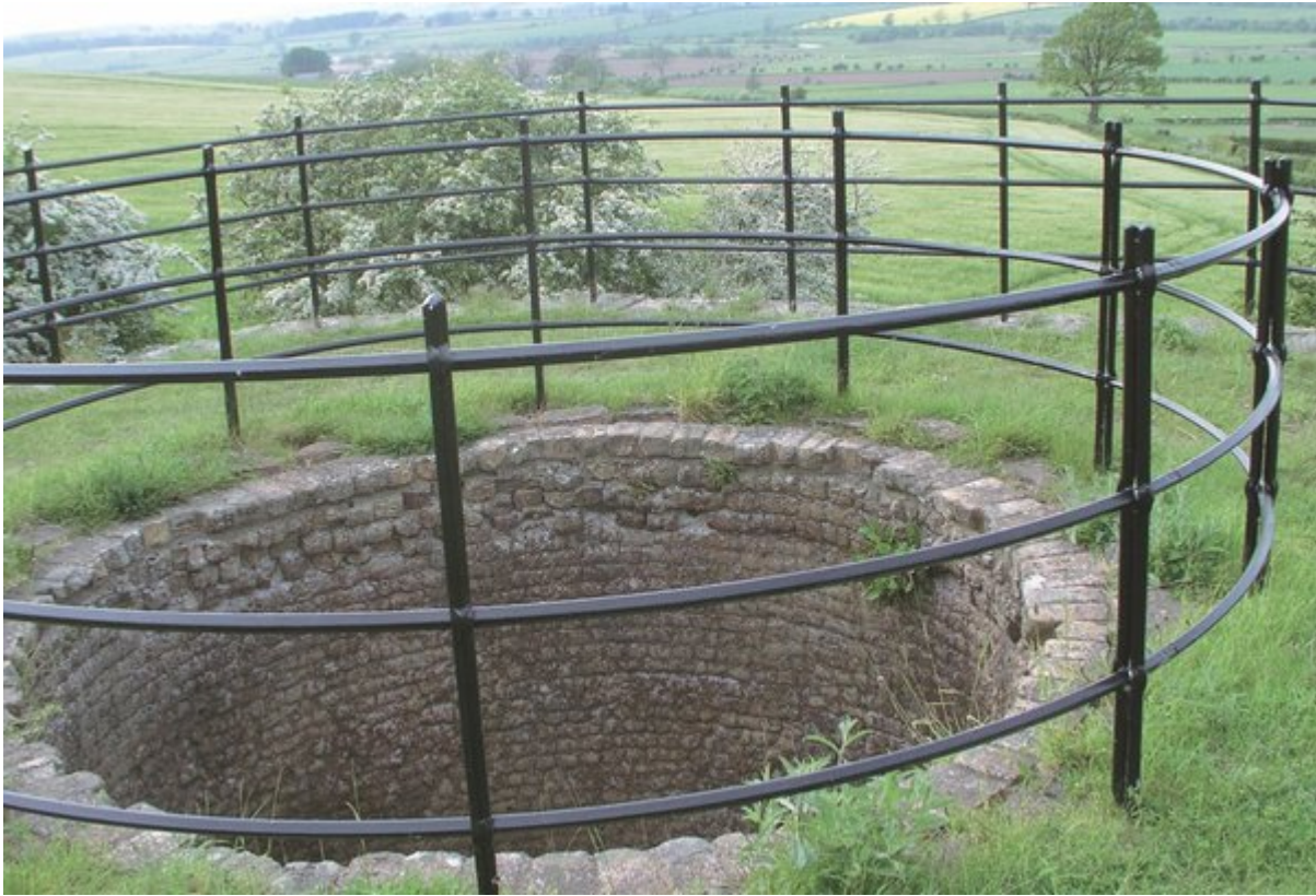
(Figure 84) The opening into the pot at Great Tosson Limekiln.
