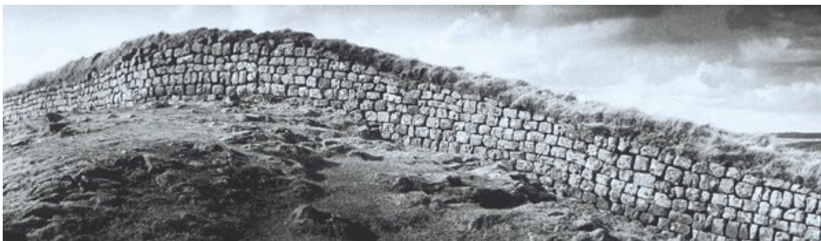
(Figure 18) Squared blocks of sandstone in Hadrian's Wall near Housesteads © Emma Amsden.
