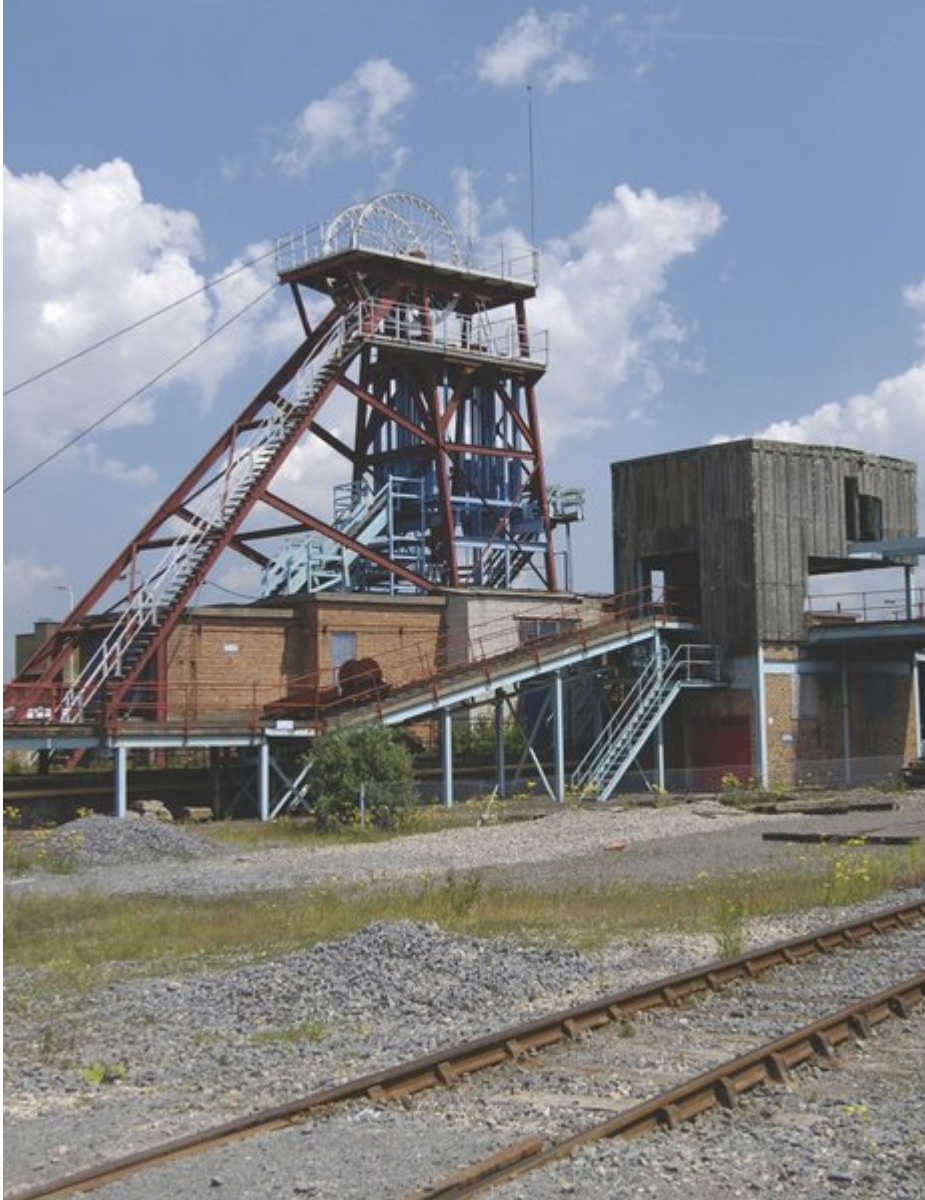
(Figure 91) The former Snibston Colliery.
