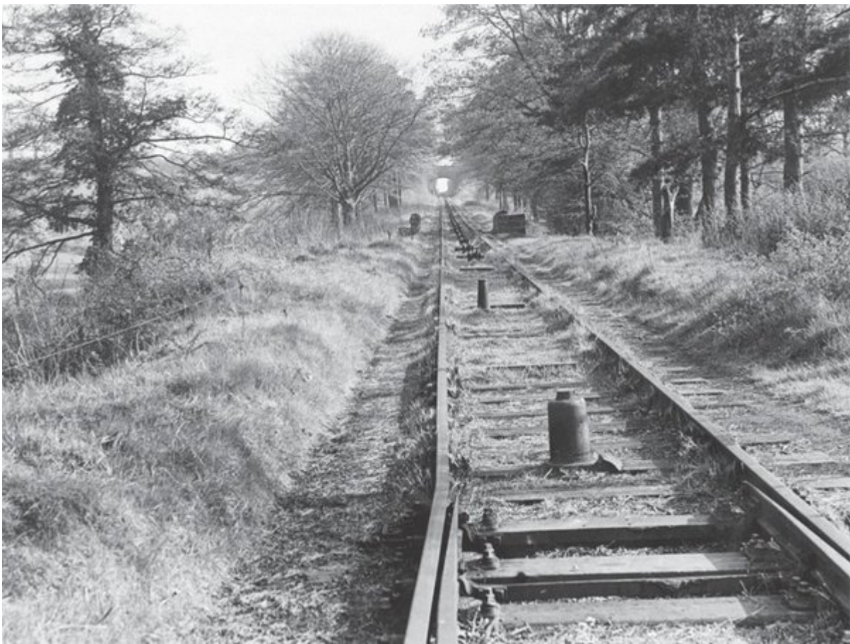
(Figure 94) Former railway line on the Swannington incline. Photographs © The National Railway Museum.
