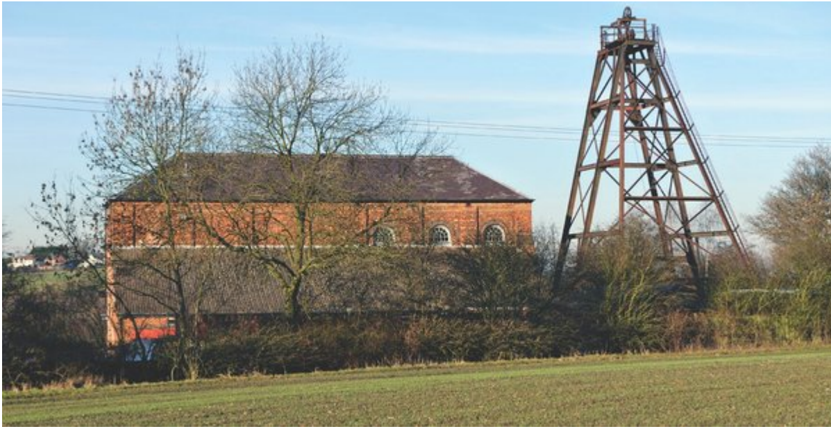
(Figure 97) Headgear of the former Calcutta Pit, Swannington. This pumped all the water out of the Leicestershire coalfield up to 1991.
