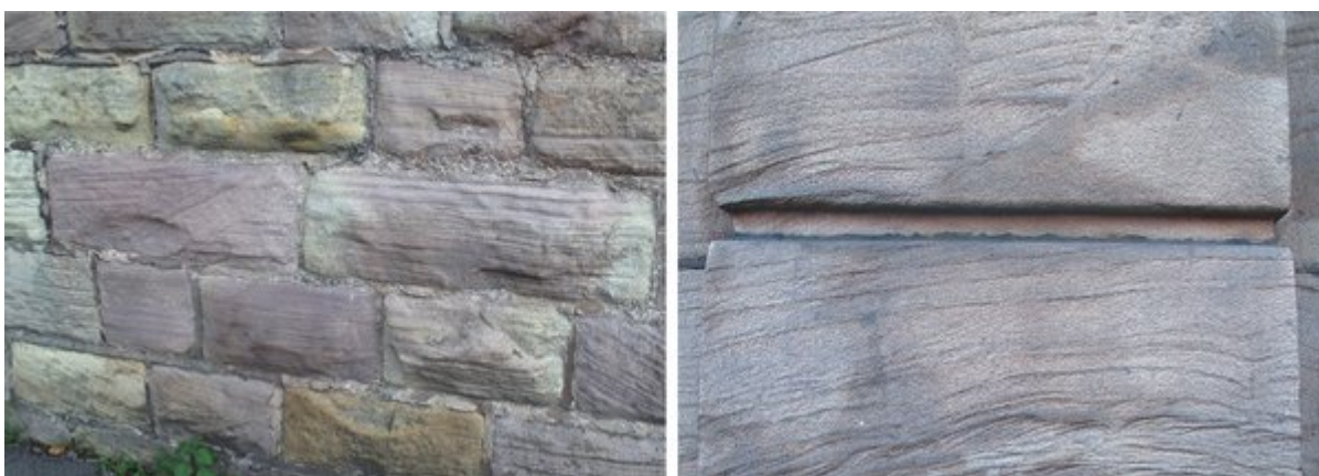
(Figure 100) Contrasting sandstone building blocks: on the left, Millstone Grit in the wall of Trent Bridge, Burton. Note the clear parallel lamination and cross-bedding (pp.8 and 10) in the blocks. On the right, finer-grained Bromsgrove Sandstone, seen in several buildings.
