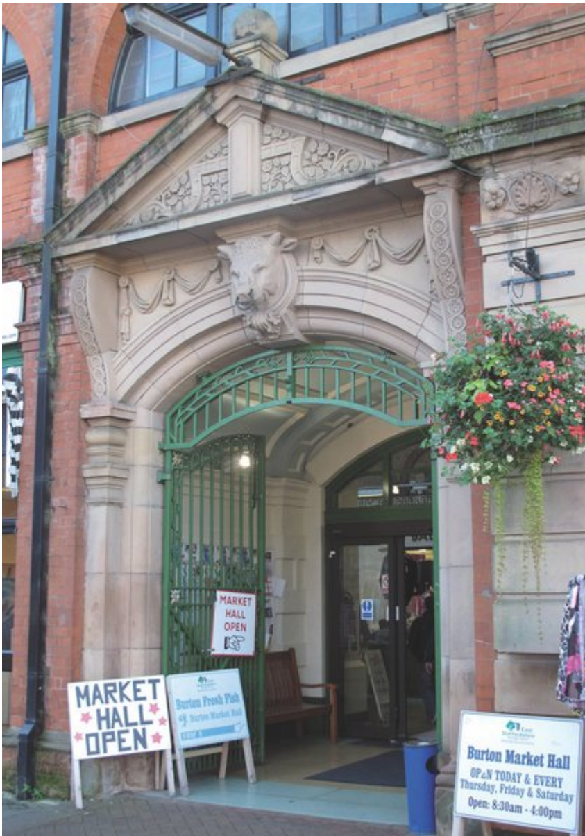
(Figure 102) Market Hall in Burton with the distinctive carved bull's head. The stone frontage is built of Millstone Grit sandstone.
