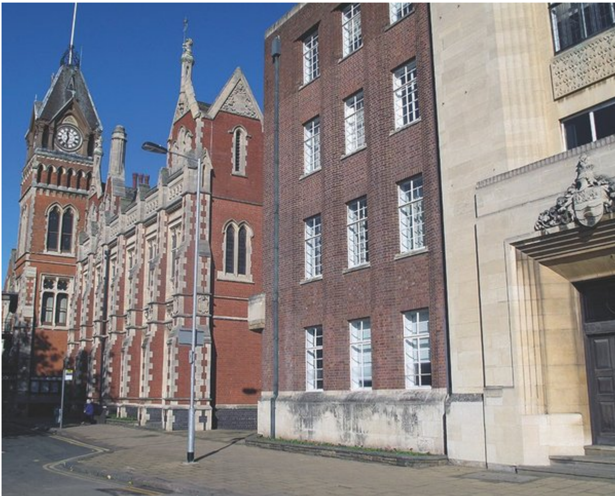
(Figure 104) The newer, yellowed Portland Stone facade of the 1938–39 municipal offices with the older Victorian (1878) Town Hall clock tower facade of pale Lincolnshire Limestone (Ancaster Stone) and red brick.
