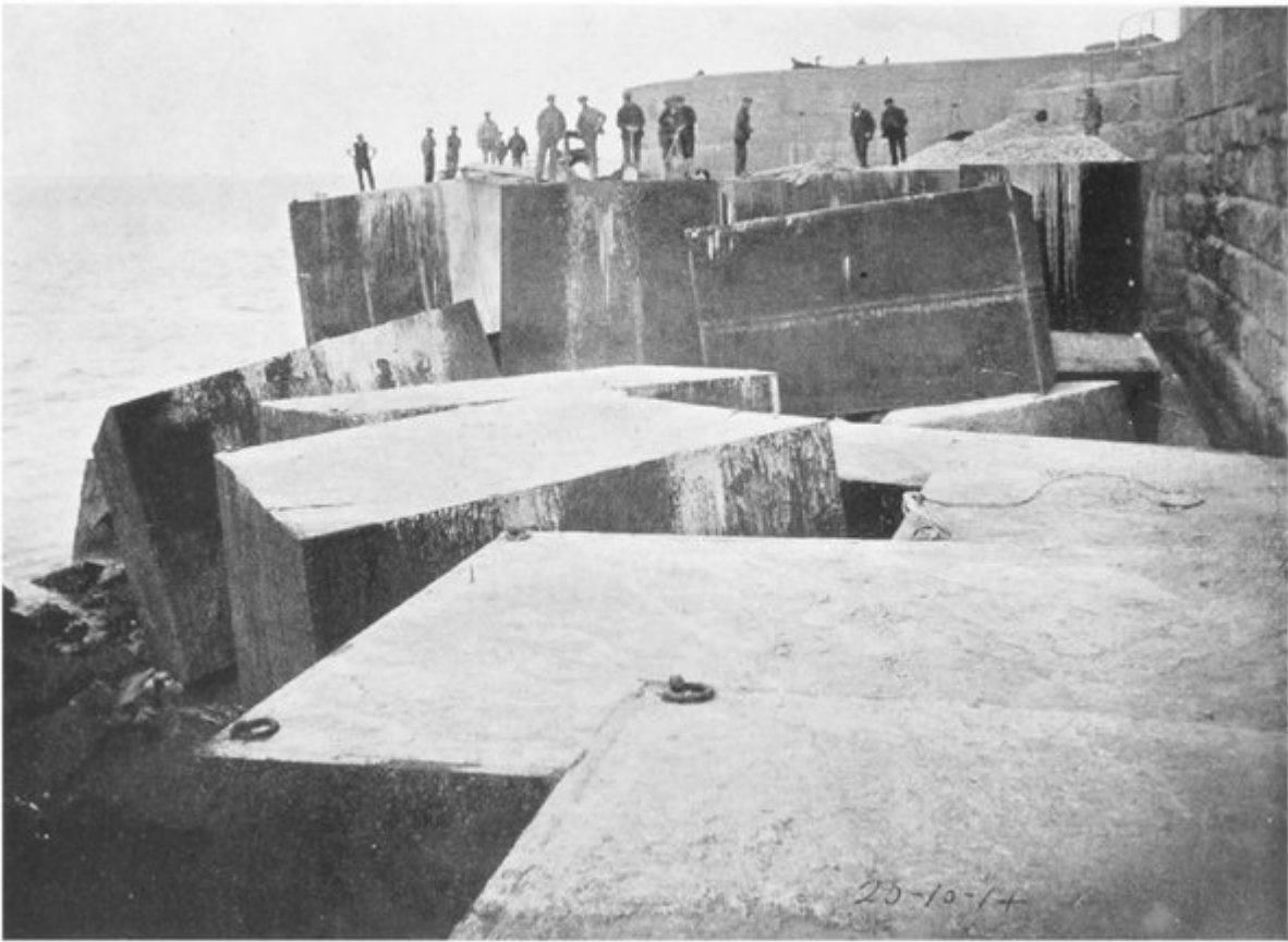
(Plate 59) Blocks moved by the Sea. Holyhead Breakwater.
