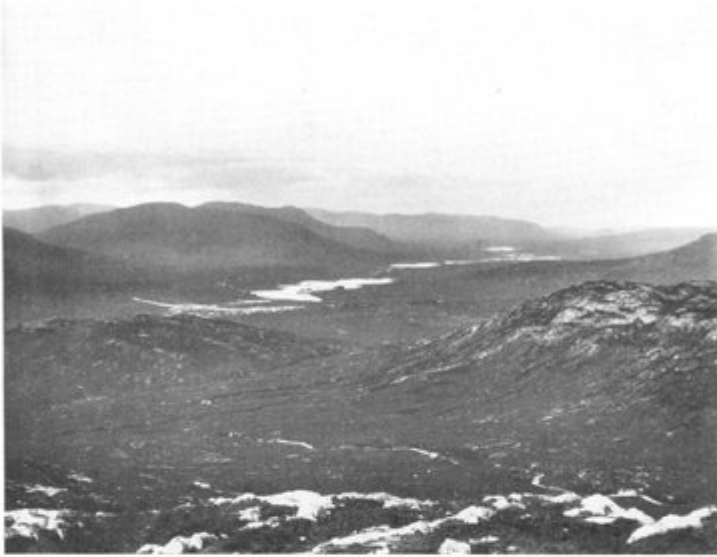
1. HANGING PORTION OF RIVER LEVEN WITH DAM SITE OF BLACKWATER RESERVOIR
