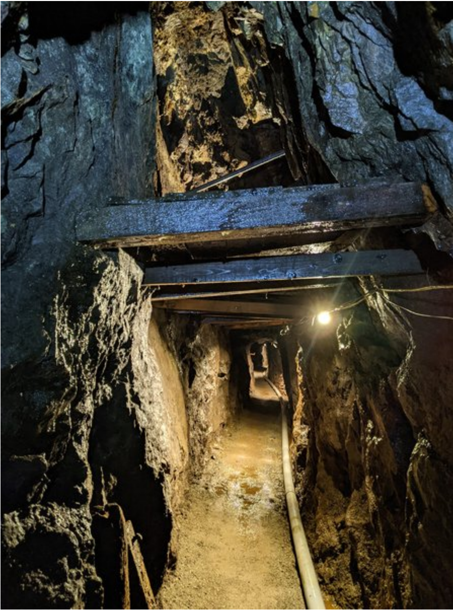
Lochnell Mine. A view underground. This mine is open to the public through the Lead Mining Museum. Copyright: Museum of Lead Mining, Wanlockhead.
